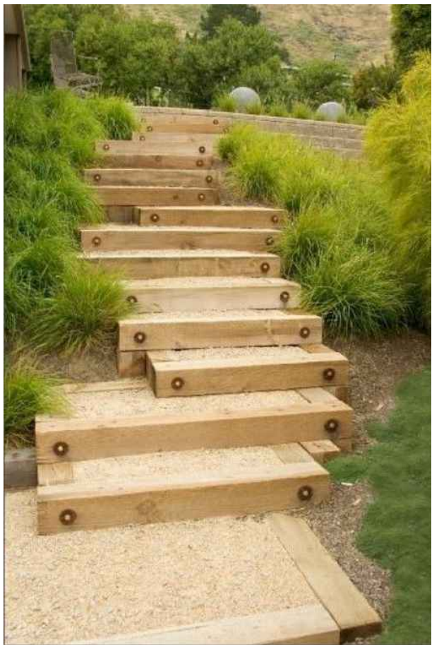
E2: Timber Edge Around Steps
